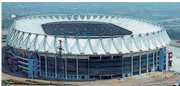
Qingdao Yizhong Stadium
