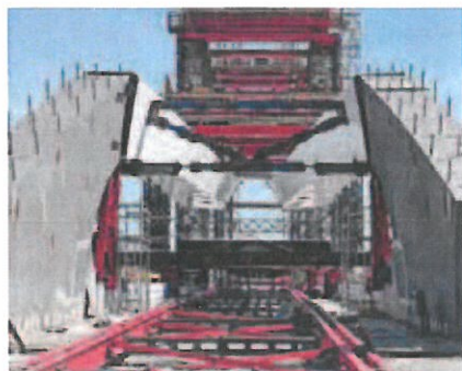
The Troja Bridge during construction.
