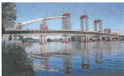
The raising of the arch during construction.
