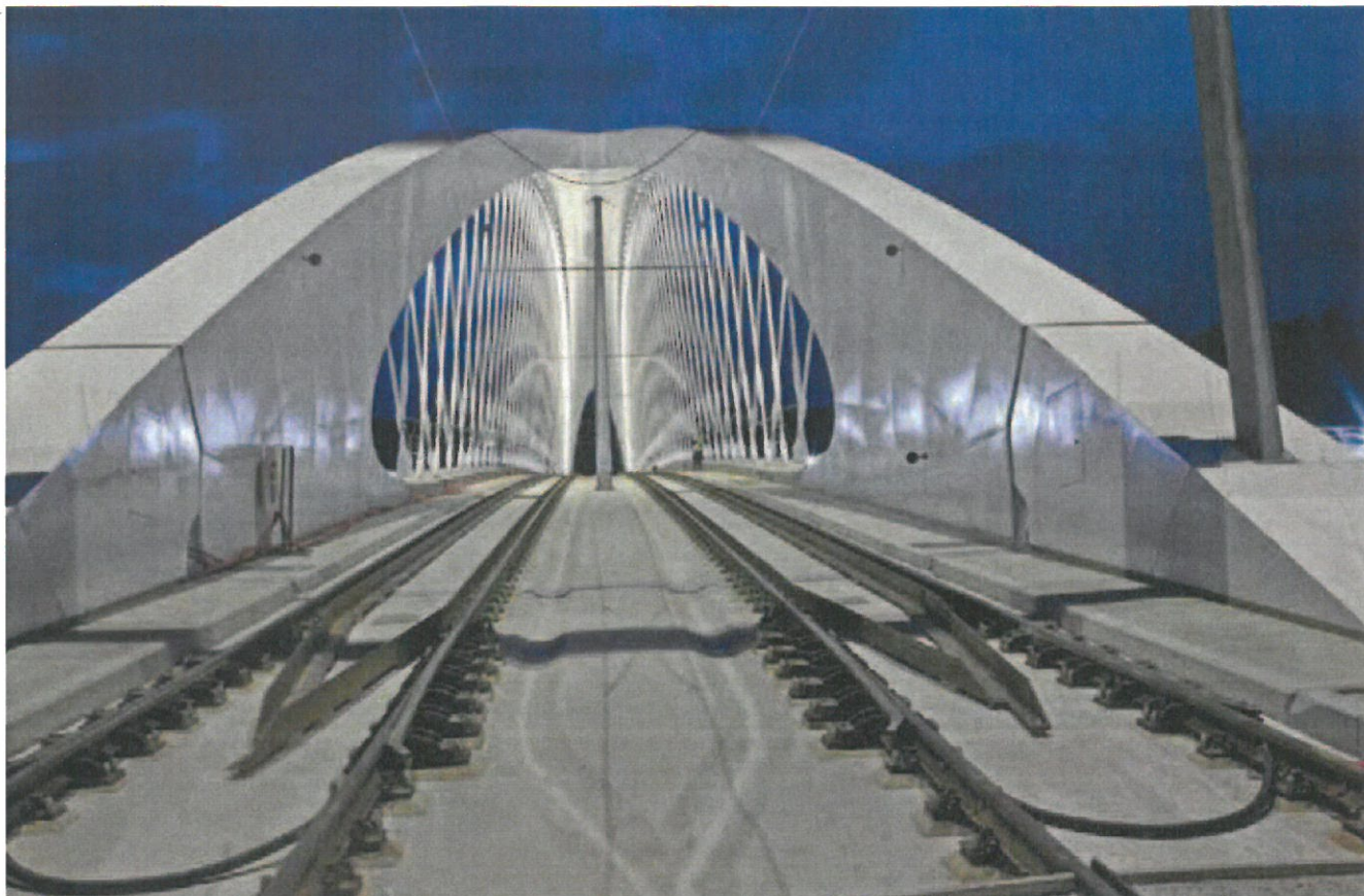
Tramway deck of the Troja Bridge.
