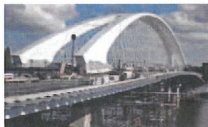
Steelwork is by Metrostav.
