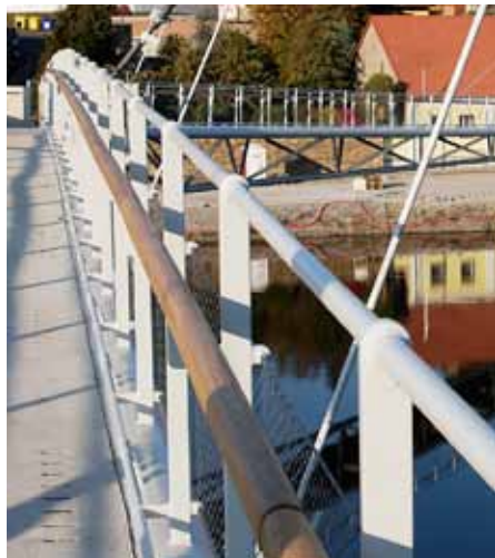
Obr. 20: Detail zábradlí a madel
