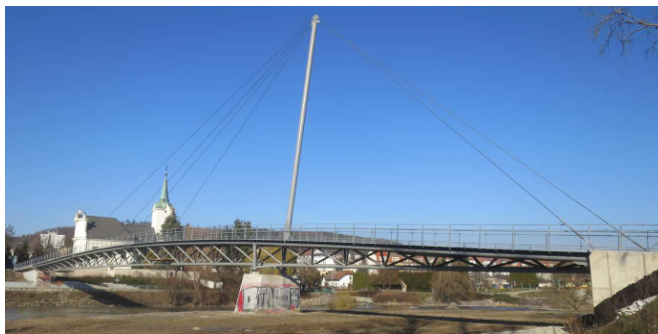
Figure 2 New triangular lattice cable-stayed footbridge
