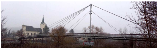
Figure 1 Original concrete footbridge
