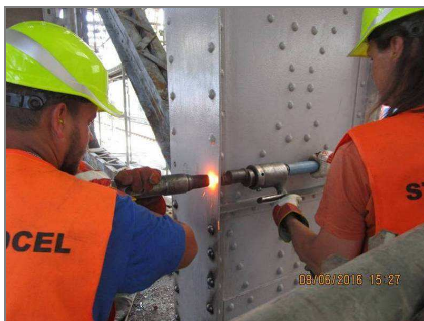
Obr. 29 Nýtování na montáži Figure 29 Riveting during installation
