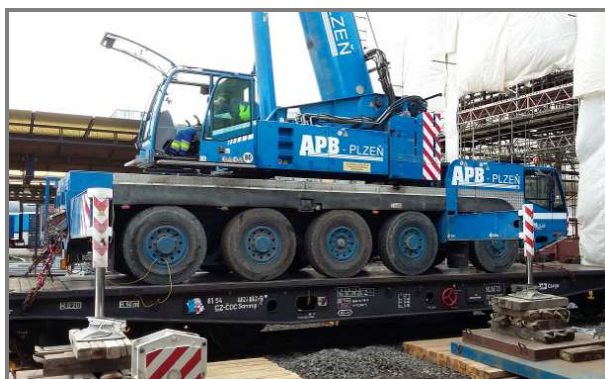
Obr. 42 Mobilní jeřáb Demag AC100 na vagónu Figure 42 Demag AC100 mobile crane on a railway carriage
