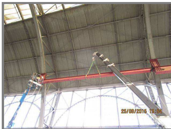
Obr. 39 Demontáž kolejnic pro pojezd lávky Figure 39 Disassembly of rails for gantry movement
